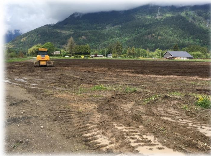
Photo 1 BGM production and placing
