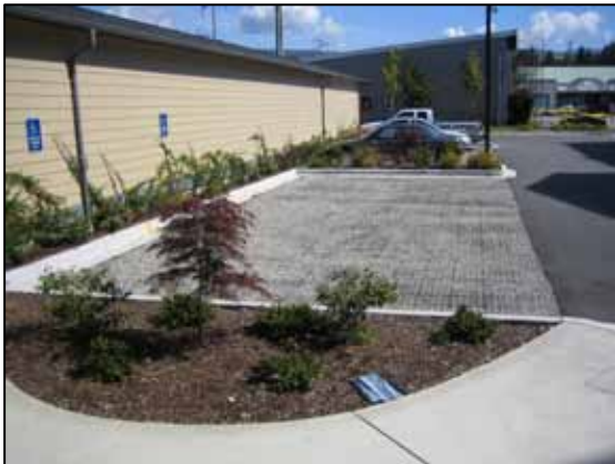
Reinforced Clean Crushed Gravel
