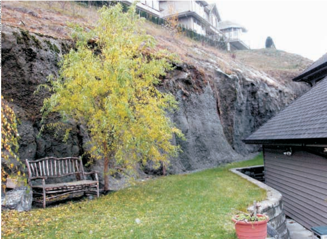
Photo 7. Sandstone face with minimal overburden on Westview Blvd.
