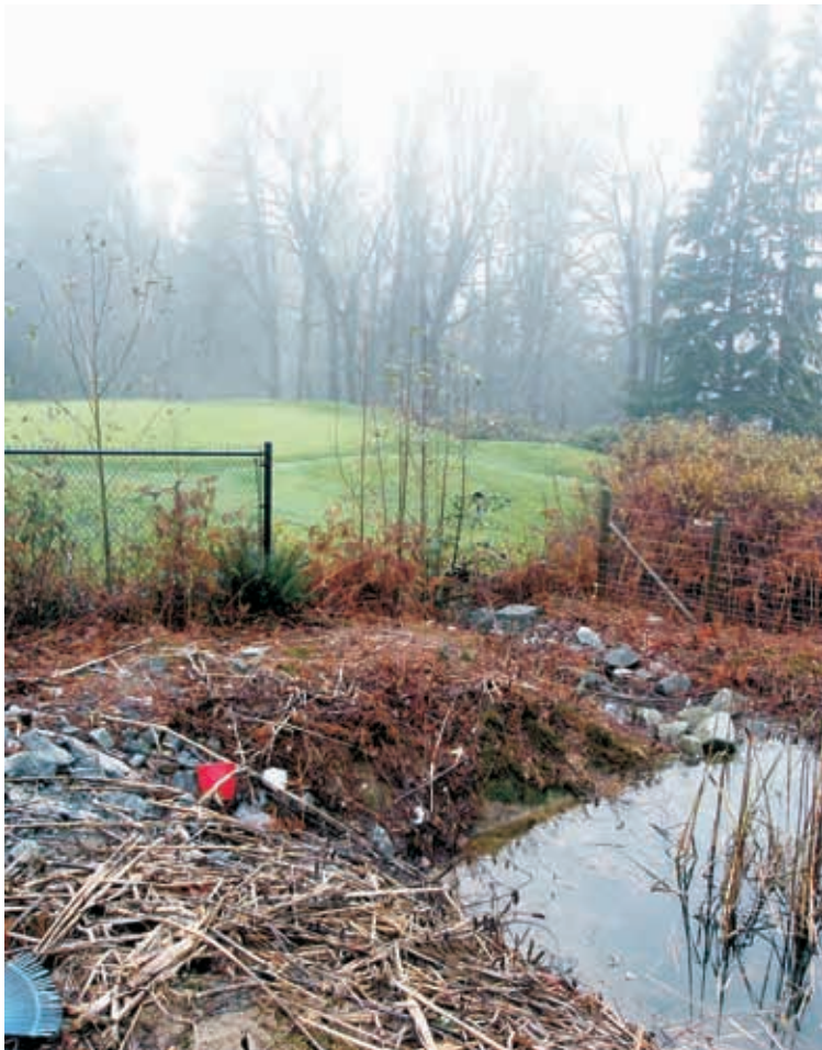
Photo 8. Soak-away pit at north end of cul-de-sac adjacent to the east of Golf Course.
