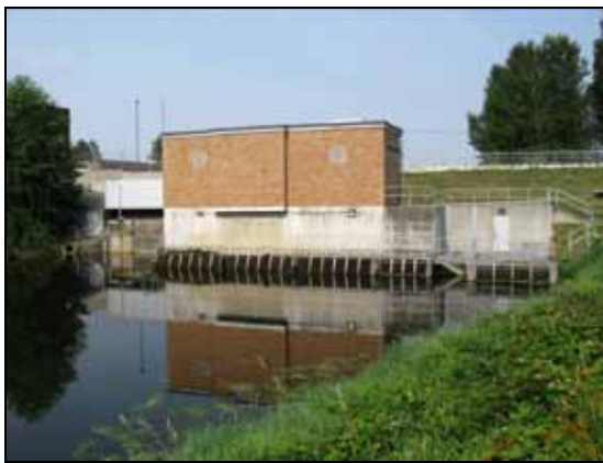
(a) Matsqui (Gladwin) Pump Station (upstream side)
