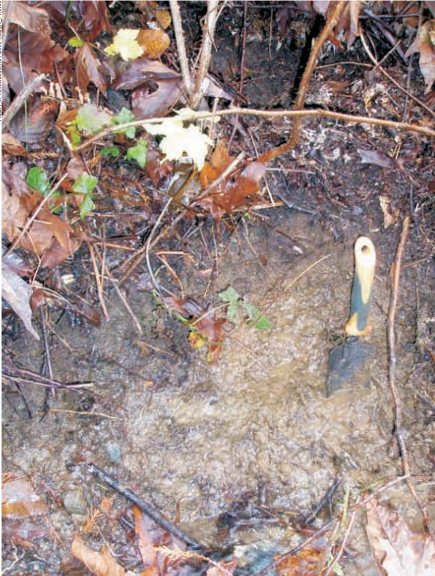
Photo 5. Saturated clayey till at Dawson Road and Charlie Spruce Place.
