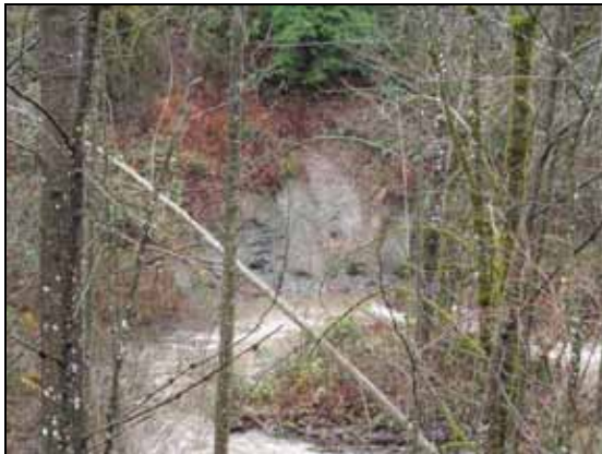
Photo 5-1: Poignant Creek Eroding Toe of Slope
