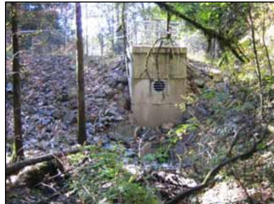
Photo 1-14: Auguston Instream Detention Facility
