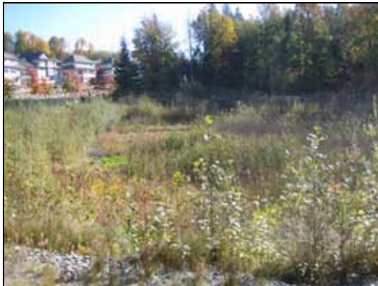
Photo 1-13: Auguston Blauson Detention Pond
