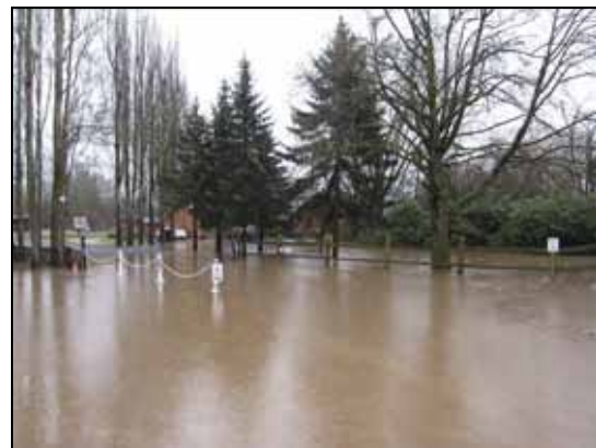
Photo 1-4: Clayburn Village Flooding of 4290 Wright Street Dec. 2010
