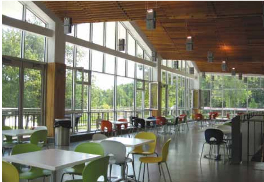
Wood was often used in modern buildings as a finish to contrast with more industrial materials, or as part of an acoustical treatment on ceilings and walls. The wood ceiling and column claddings of the Beaver Lake Pavilion in Montreal were carefully preserved as part of the recent rehabilitation of the pavilion.
