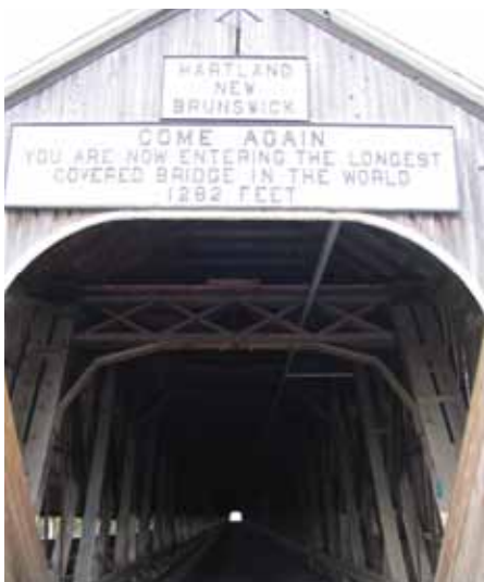
The Hartland Covered Bridge, crossing the St. John River at Hartland, NB, is the world's longest covered bridge. It is significant for its structural qualities, contributions to transportation and as a symbol of the heritage of covered bridges in New Brunswick. The present bridge is a standard covered bridge structure composed of a Howe truss superstructure enclosed with vertical unpainted weatherboard siding. When the New Brunswick Department of Transportation recently rehabilitated the bridge by installing a fire suppression system, care was taken to ensure that this new system was barely visible in the upper structural system.
