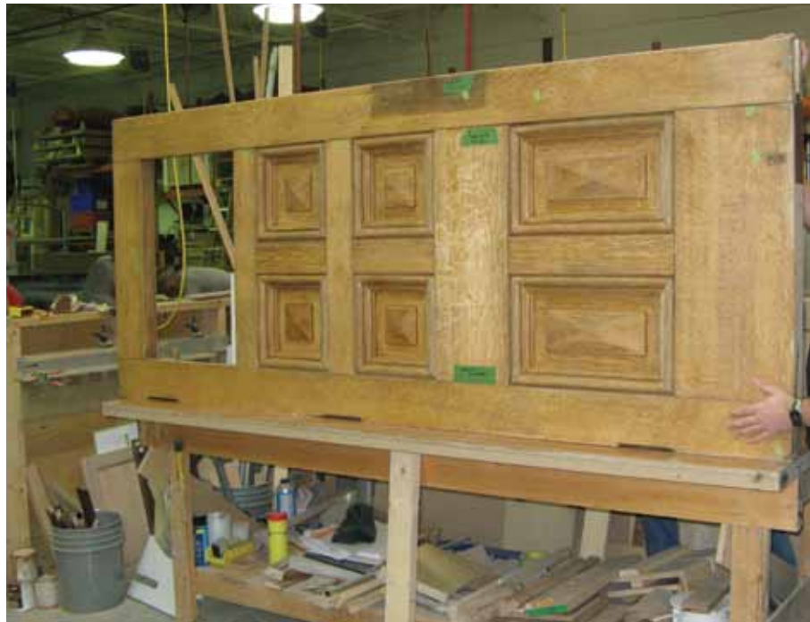
Preserving the wood doors of the Langevin Block in Ottawa included carefully dismantling the doors to permit the damaged and decayed wood to be repaired.
