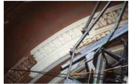
When restoring decorative plaster in the Walker Theatre in Winnipeg, moulds were made of existing plaster elements. The deteriorated plaster was then patched and repaired using the moulds to match the original.
