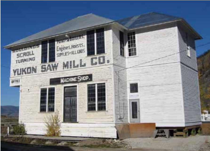
A compatible addition to the rear of the Yukon Sawmill Co. Office provides space for services. If necessary, it could be removed without affecting the building's historic fabric. One window opening and the surrounding wall framing were altered to provide space for a connecting door.
