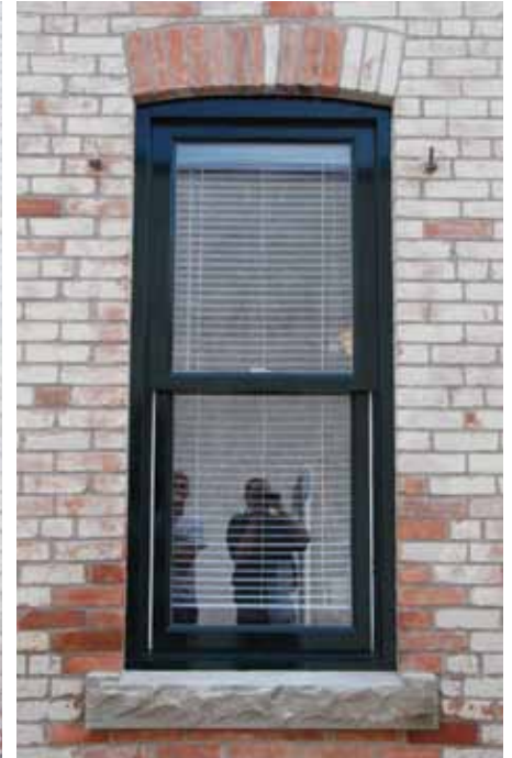
Left: North façade window prior to rehabilitation showing eroded mortar joints, cracking due to frost action within the wet wall, and delamination of the sandstone sill.
