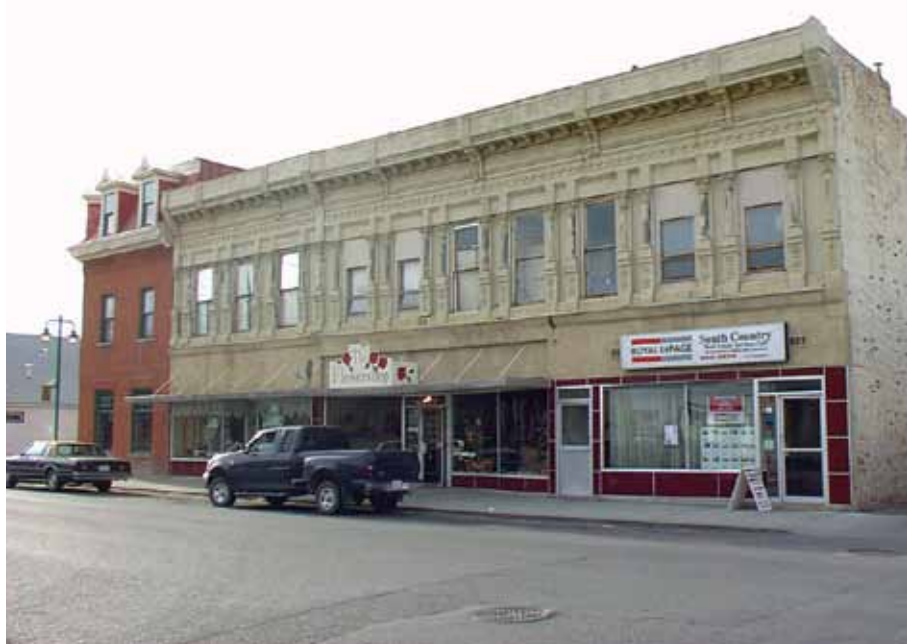
Before rehabilitation: east façade, looking southwest.
