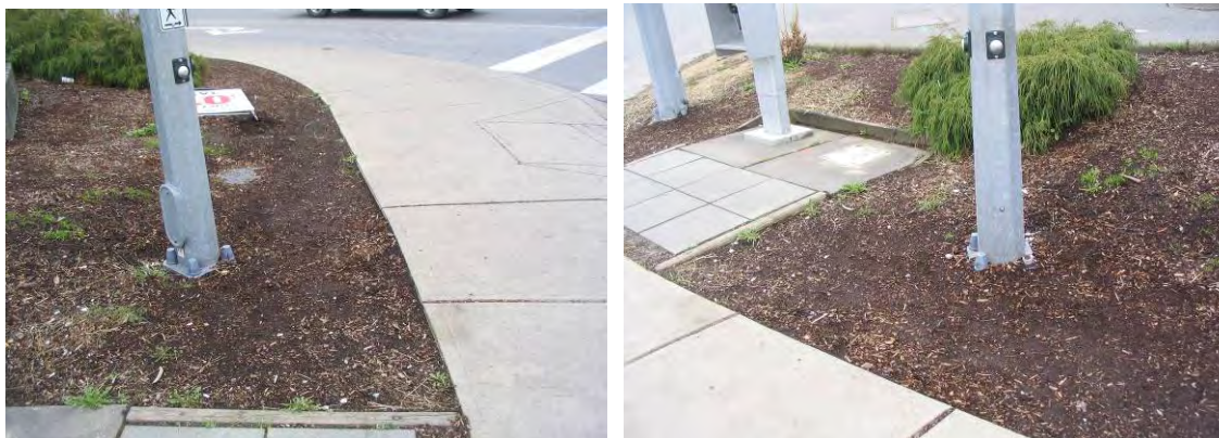
Figure 60: Difficult to access button on poles at crosswalk. Soft and muddy surface around pole. Scooter may get stuck on soft surface.
