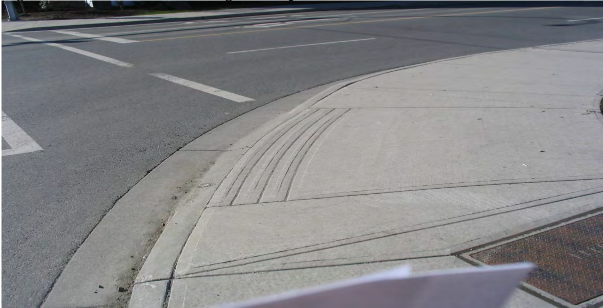
Figure 76: Wide curb cut with a gentle slope and smooth surface.
