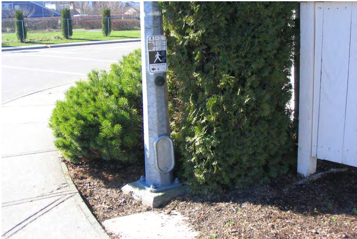
Figure 71: Crosswalks: Buttons on pole difficult to access.
