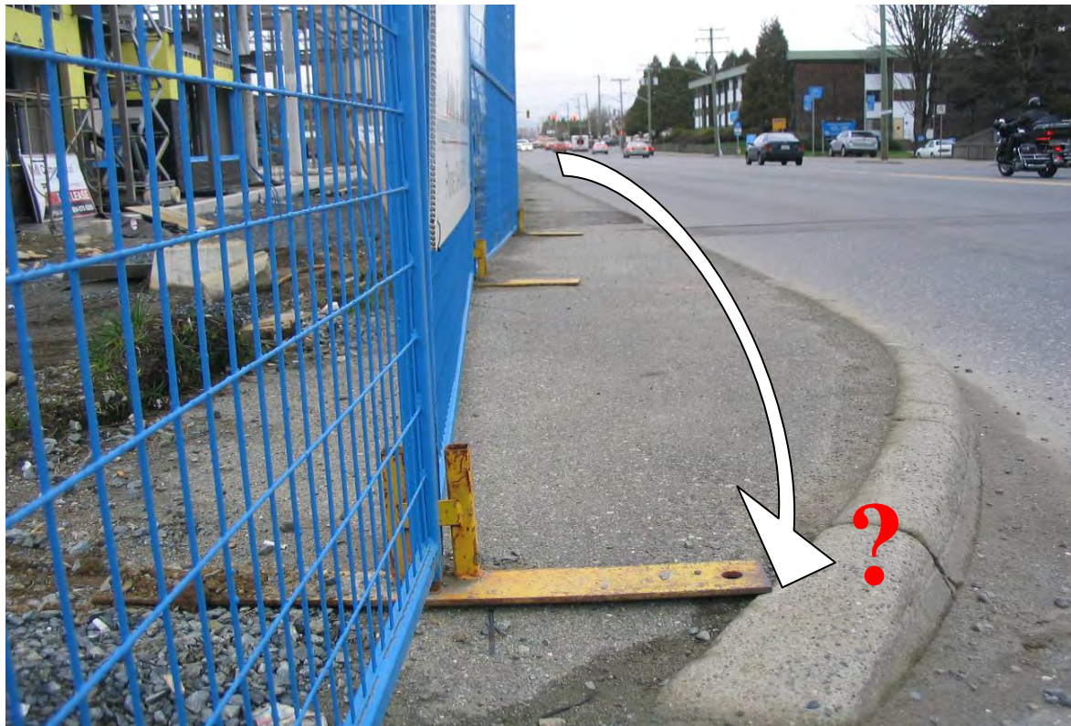
Figure 57: Access point to sidewalk on overpass bridge: Sharp and uneven edge.
