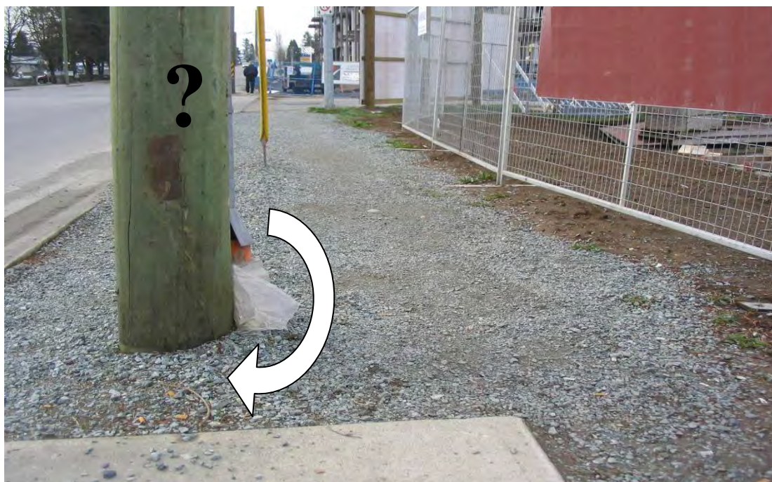
Figure 53: Construction Site: Change in surfaces. Sidewalk comes to an abrupt end, change to uneven gravel.
