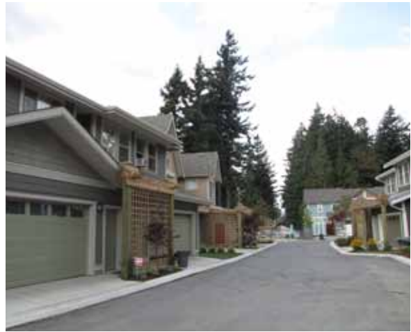
Figure 9. In this back alley, overlook from second storey windows provide opportunities for natural surveillance and privacy screens are visually permeable.
