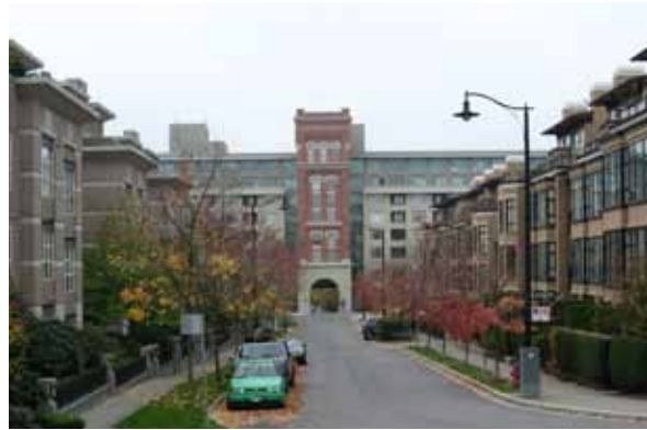
Figure 4. Site buildings to define public open spaces. Site buildings and provide distinctive architectural features to terminate a street end view.
