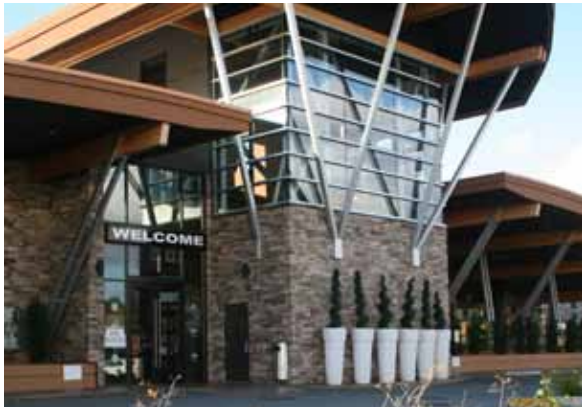
Figure 17. When a blank wall is unavoidable, devices such as planters can break up the visual impact and minimize opportunities for vandalism.
