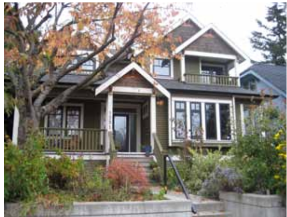
Figure 7. The transition from public to private is marked by design cues: a semi elevated entryway, landscaping, and a front porch help to define territory in a way that preserves privacy and supports a sense of ownership yet still allows for natural surveillance.
