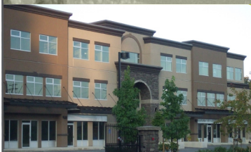
City Scape Building
