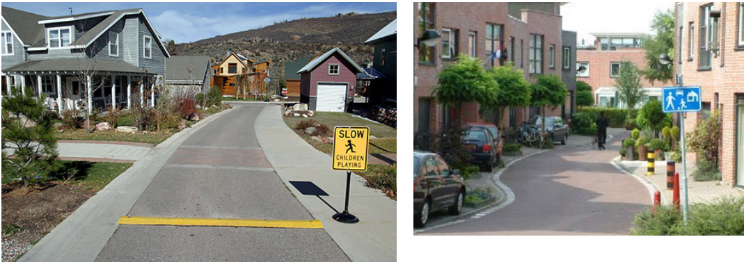
Figure 15. Woonerf's implement traffic calming measures and signage to inform the public of the type of street they are entering. http://streetswiki.wikispaces.com/Woonerf
