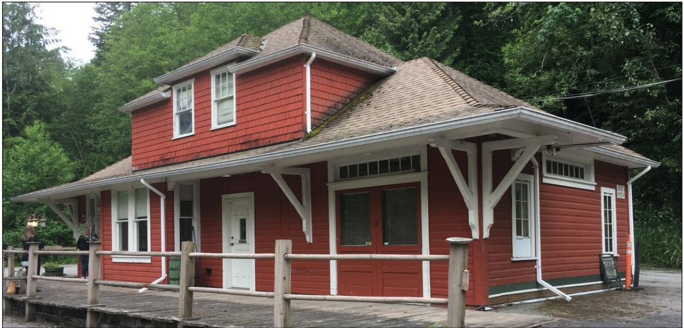
Figure 6 – C.P. Rail Station
