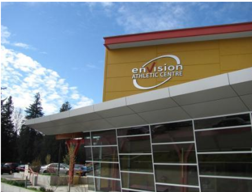
UFV - Abbotsford Campus Recreational Facility
