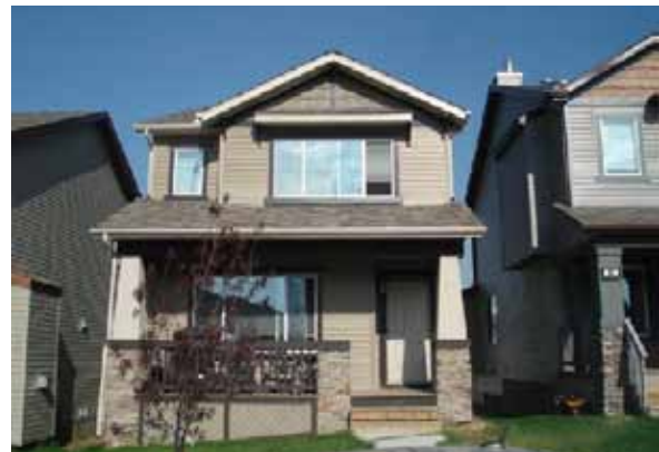
Figure 30. An example of a single family home with a positive relationship to the street.
