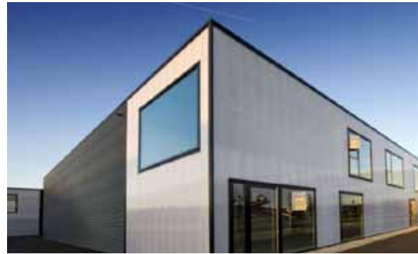
Figure 25. Windows in the lobby, internal corridors and above ground level.
