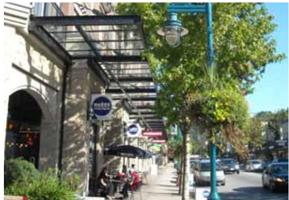
Figure 23. Recessed entries, glazing, weather protection and ornamentation create a welcoming frontage without creating blindspots.
